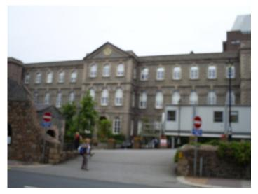
The walls are of solid construction, with a tiled un-insulated pitched roof, solid un-insulated floors and it is mostly double glazed. There is a single lift in the Block, which is in the process of being upgraded.
