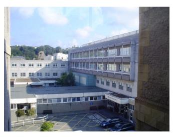
The walls are believed to be of narrow empty cavity construction, with a flat un-insulated roof, solid un-insulated floors and it is mostly single glazed. Much of the ground floor has louvred opening sections within the glazing, which results in excessive uncontrolled ventilation during the heating season and unacceptably high heat losses. There is a single lift in the Block, which has been recently upgraded.
